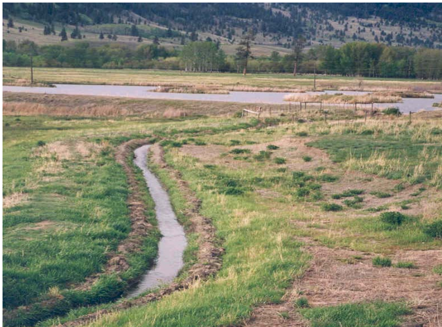
Figure 4.10 Open ditch conveying water at Nicola Lake.
